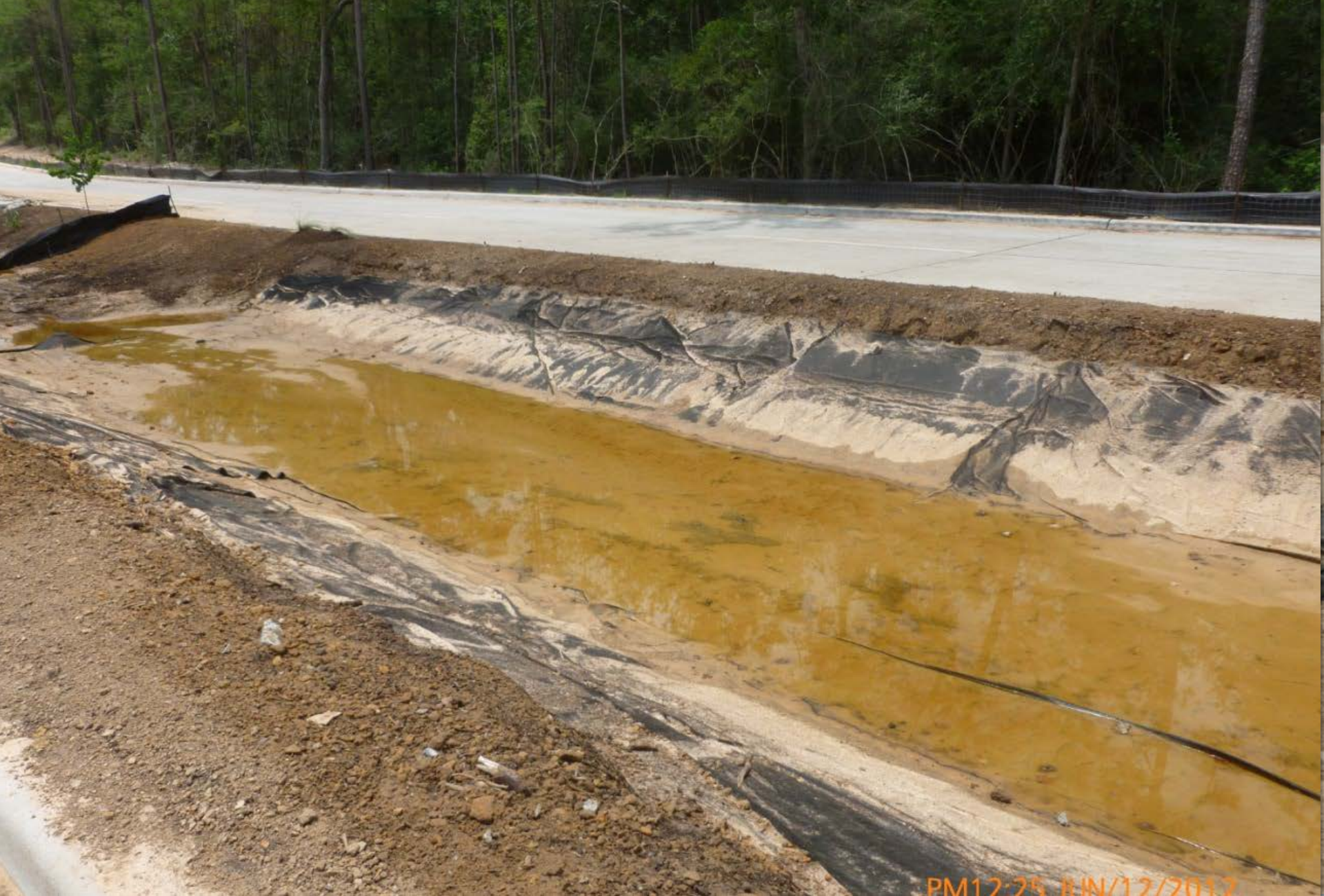
Construction Issues: Erosion Control
