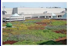
the growing media and plantings. Rainwater is retained until the assembly is completely saturated, and excess water is
