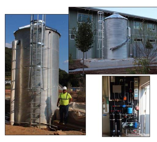
Harvesting rainwater from roof to use for **toilets and irrigation**
